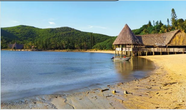
Photo 1. Covered dock, made with wooden poles in radiata pine ( Pinus insignis ) treated with CCA (Chromated Copper Arsenate), Nouméa, New Caledonia, France. Photo K. Candelier.
