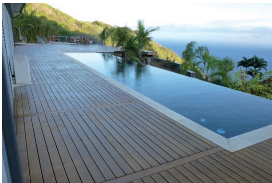
Decking around an infinity pool – By Agencement Tiby, supplies from Fibres Industries Bois , La Réunion, France. Photo David Bodelu, Fibres Industries Bois .
