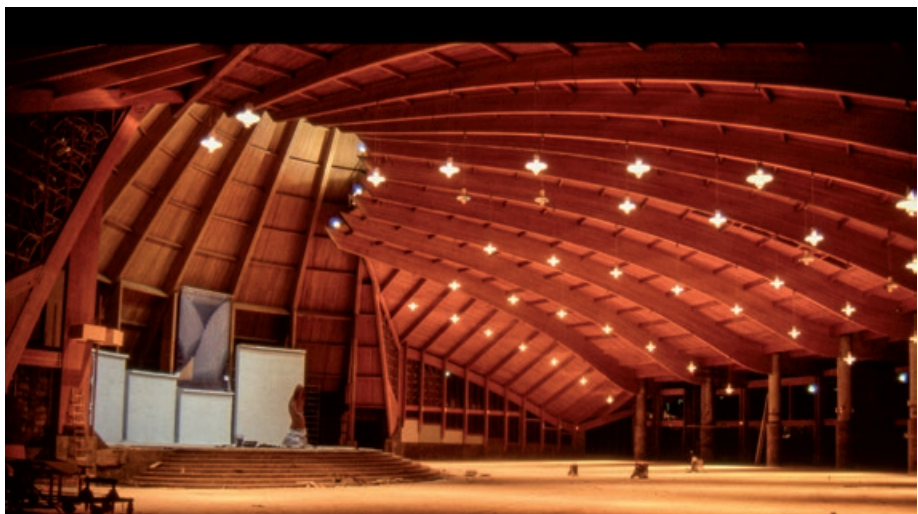
Glued laminated indoor structure at the Mary Queen of the Apostles Basilica in Yaoundé (Cameroon). Photo J. Uhalde, UBC.
