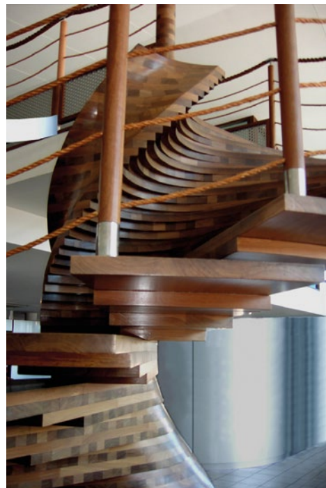
Interior staircase in glued laminated timber – by Les Bois du Pacifique, Nouméa (New Caledonia). Photo J. Gérard, D. Guibal, Cirad.
