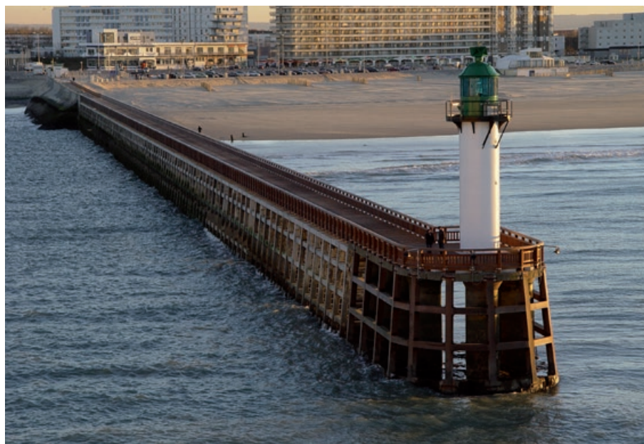
“Tillac” on the Calais pier – Design by Bois et Loisirs(France). Photo D. Delequeuche.
