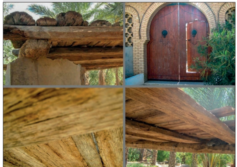
Figure 2. Date Palm stems, treated naturally by salt waters of the Lake of Chot Djérid used as structural materials in the region of Djérid in Tunisia.
