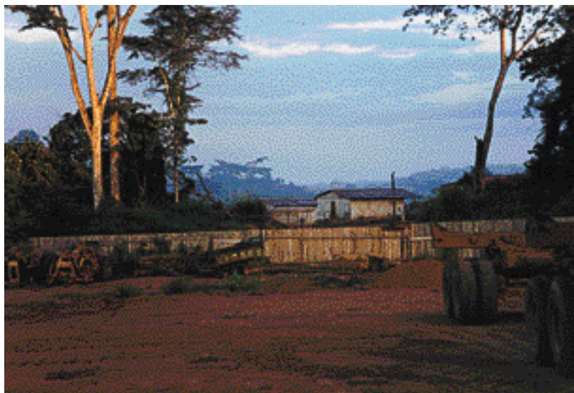
Photo 7. Palissade entourant un point franc industriel. Ce statut juridique étant destiné à favoriser l'industrialisation. Fence surrounding an industrial free zone. This legal status being designed to encourage industrialization.
