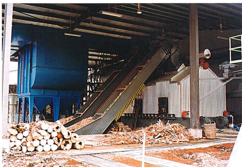
Wood-based cogeneration unit in an industrial complex in Malaysia.
