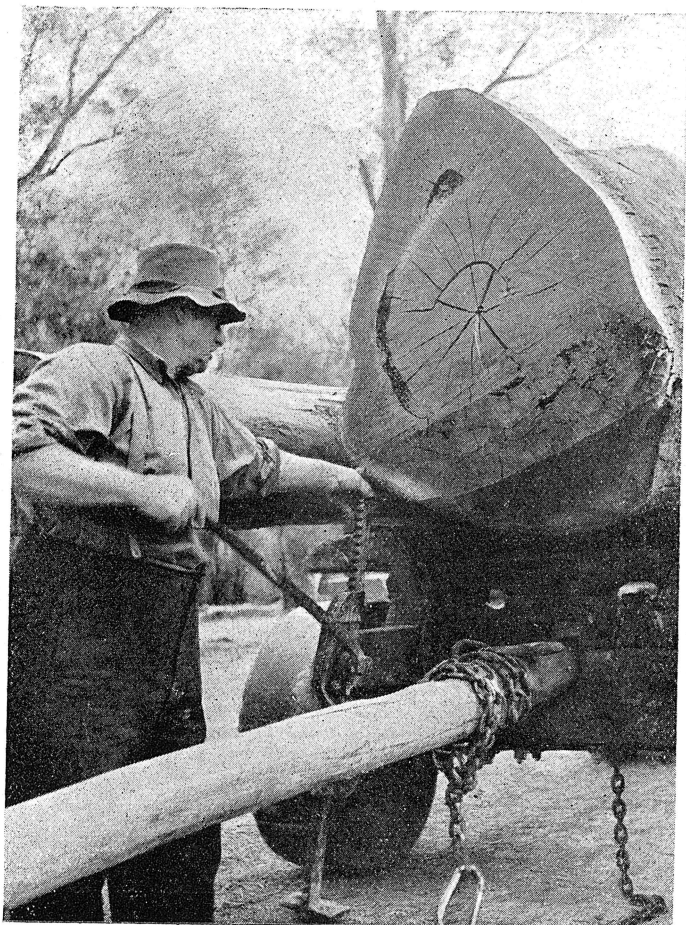
On arrival at the river-side log landing, the teamster uses a jack to roll the logs off the jinker.
